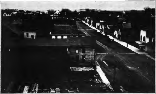
BIRD'S-EYE VIEW OF BENNETT FROM THE SOUTH
